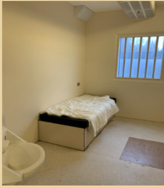
Separation unit cell at the Harmondsworth IRC
